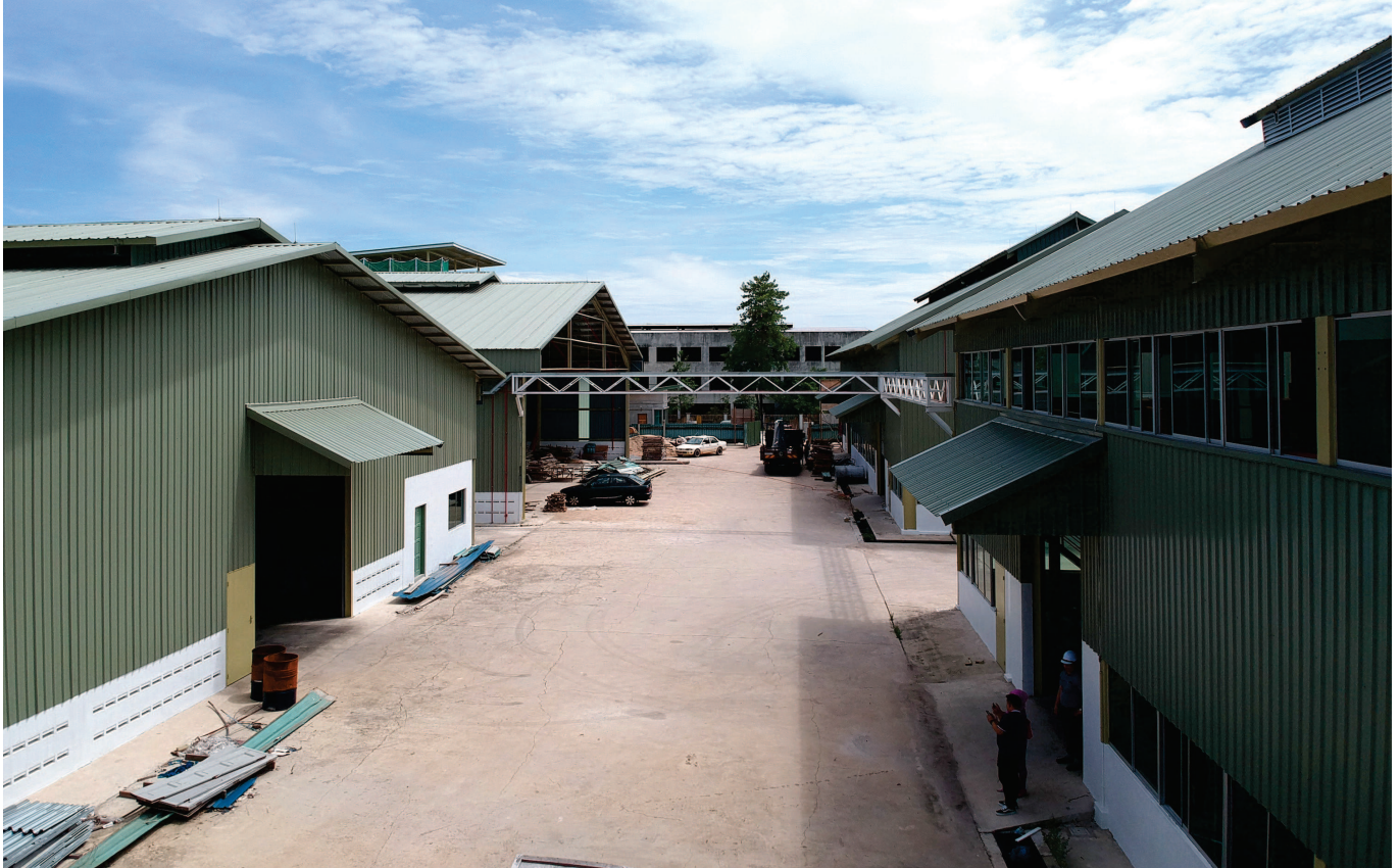
Yung Chi Paint Factory, Kawasan Perindustrian Bukit Rambai, Melaka.
